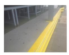
28E ARCTEC has also been used on a pedestrian loading platform at a UK airport, as part of its drive to prevent trips and slips in the workplace. The airport has chosen 28E to replace the current chequer plate surface to improve grip, particularly in the wet. As this is also an external application the platform was arcsprayed with 100 microns of aluminium before being coated with 28E.
